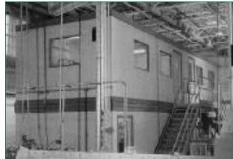
Non-combustible steel construction enables the NCP-1000 to be placed in areas where combustible construction is not allowed
